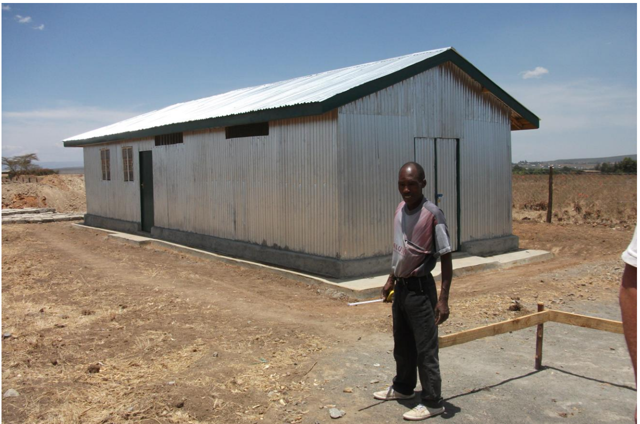
Site foreman outside his office, store and caretakers house
